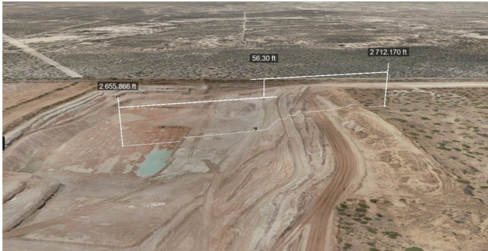
Figure 13.1: Active Quarry Face at the Crane Operations
