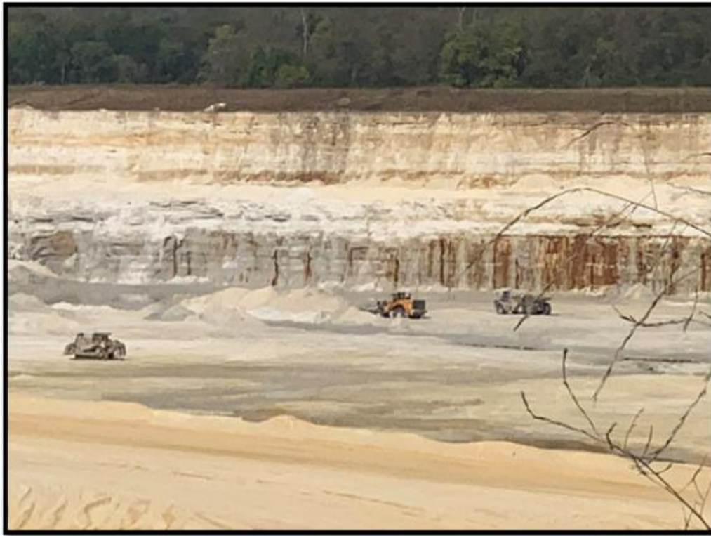
Figure 13.1 - An overview of the sandstone mining operations at the U.S. Silica Ottawa Site showing the St. Peter sandstone face and pit loading and hauling.
