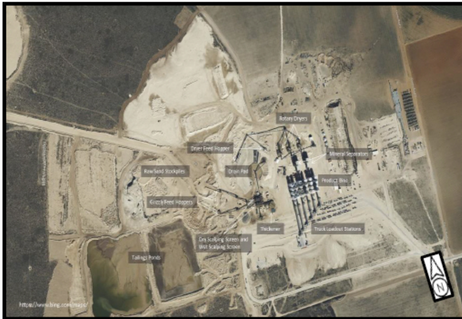
Figure 14.1 Aerial photo of the Lamesa, TX U.S. Silica plant.
